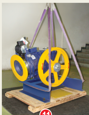
Tighten The Lifting Belt Before Remove Traction Machine From Channels
