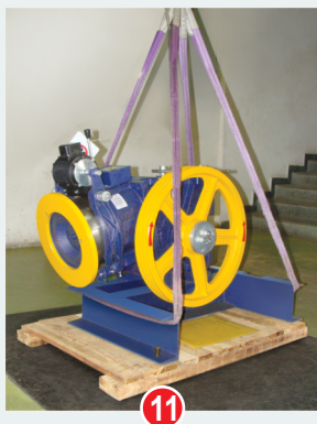
11 Tighten The Lifting Belt Before Remove Traction Machine From Channels
