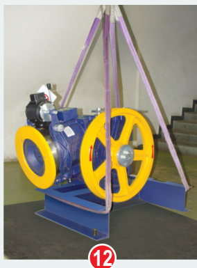
12 Lift Traction Machine & Put In Machine Room
